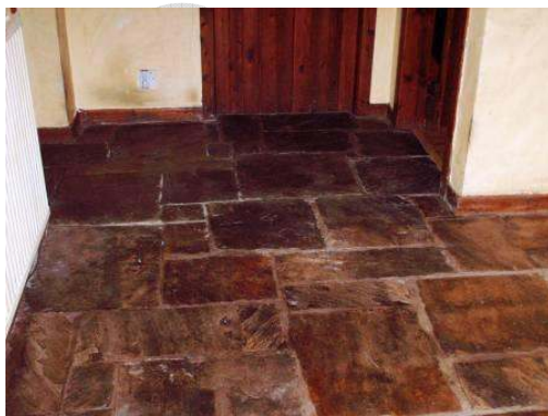
Picture shows how the sealer has brought out the colour in the Sandstone.
