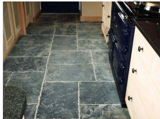
Picture shows slate before cleaning and sealing.
