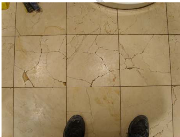
Carrera Marfil Polished Marble, with badly broken Tiles in Bathroom.
