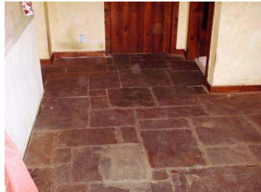
Picture shows Sandstone before cleaning and sealing.
