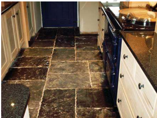
Picture shows how the sealer has brought out the colour in the slate.
