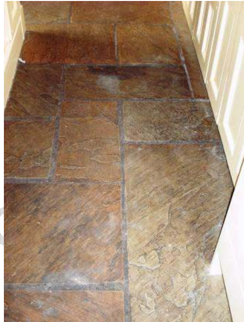
Picture shows Sandstone before cleaning and sealing.
