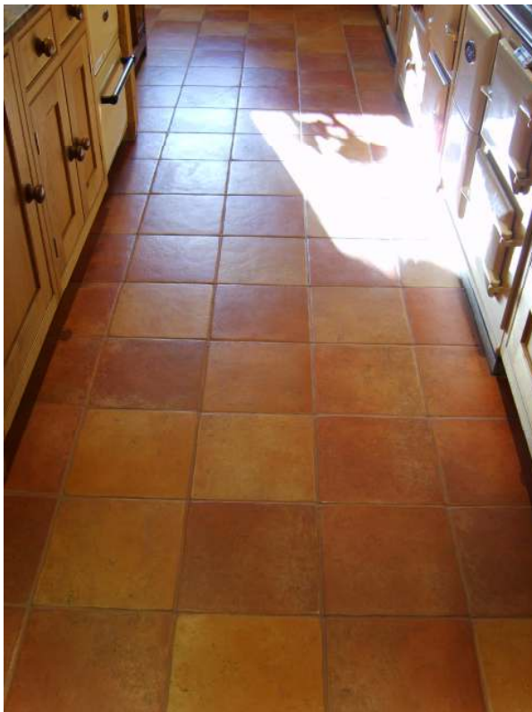
Before Cleaning and Grout Colouring
