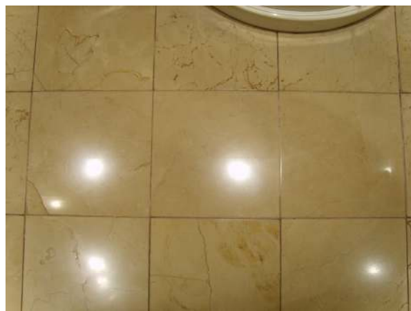
Carrera Marfil Polished Marble, with badly broken Tiles in Bathroom.
