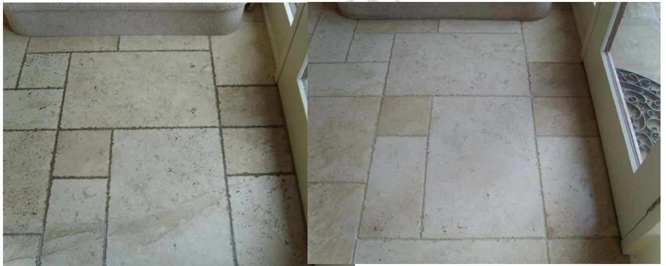
Above and below Pictures of a Chipped Edge Travertine before Cleaning with a Black Buffing pad and some Pro-clean, then sealed with 2 coats of Ultra-seal.
